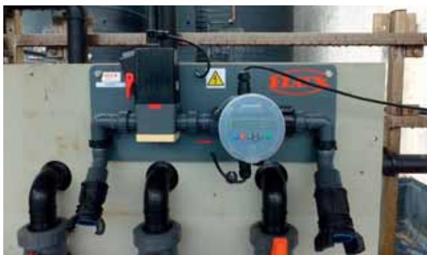
FMC 100 with switching amplifier FSV 100 installed in pipeline for semi-automatic filling.
